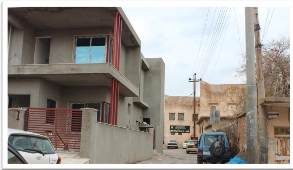
Figure 6: shows the constructing modern house in the heritage area.
