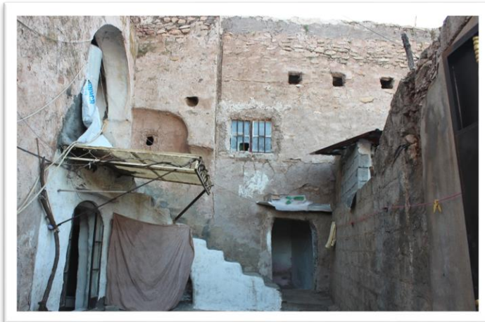
Figure 8: shows the new-constructing adding to the old part of the building. Source: author (2019)
